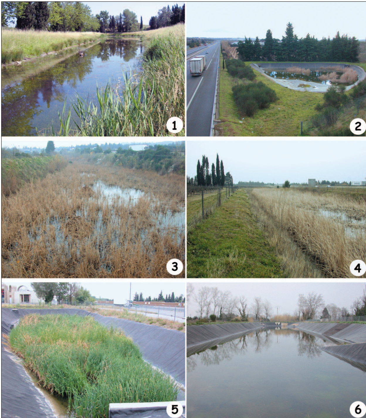
Fig. 2: Surveyed highway stormwater detention ponds with (1) ORA, (2) MRA, (3) MRB, (4) MRC, (5) SAL and (6) GRA
